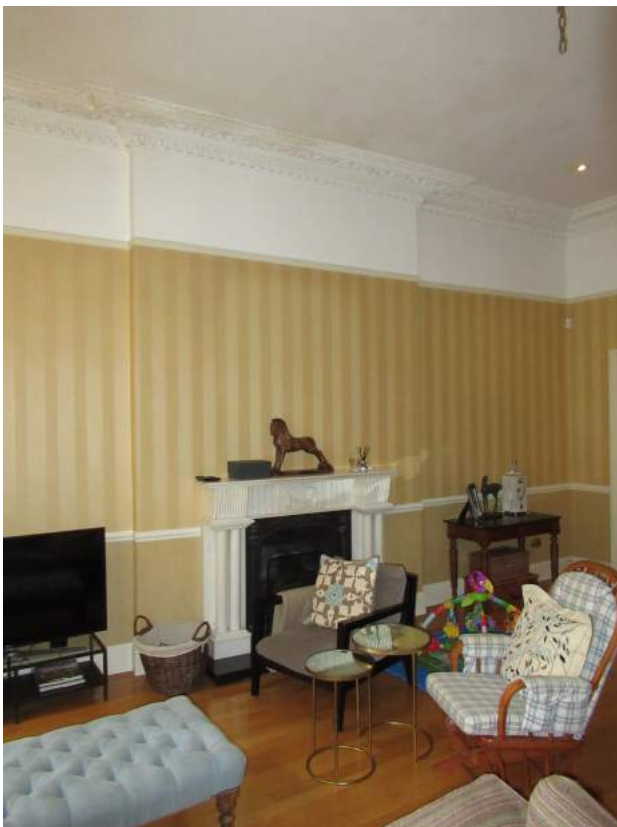
Plate No. 21. Detail internal view showing the fireplace in the sitting room in the southern half of the original house. Like its northern counterpart, this room has retained its mid-19 th century joinery, plaster coving and white marble chimneypiece.
