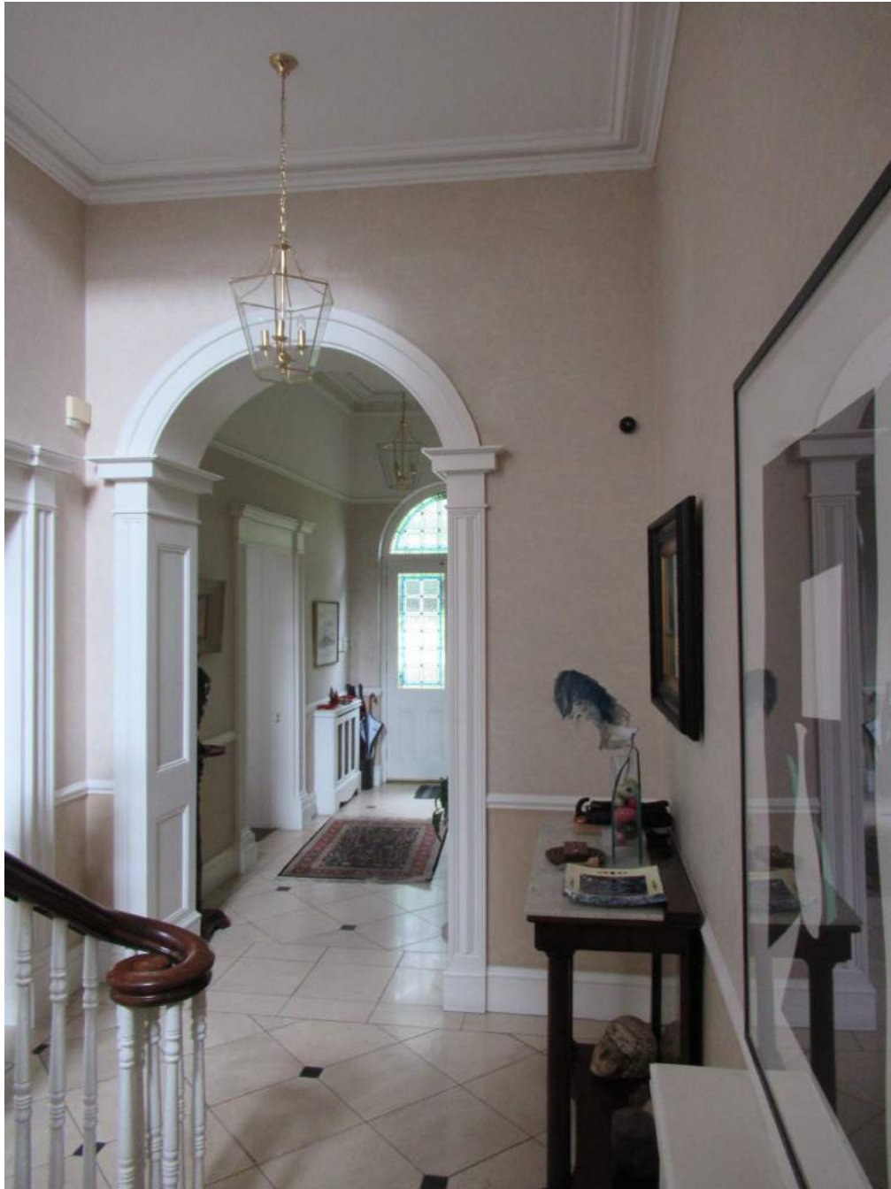
Plate No. 14. Internal view in the ground floor stairwell in the northern half of the original structure. It is believed that most of the features seen in this view date from the ca. 1860 reconstruction of the house. The glazed entrance door and transom date from the ca. 1930 division of the house into two separate properties. The floor tiles date from ca. 2000 when the northern half of the house was extended and refurbished.
