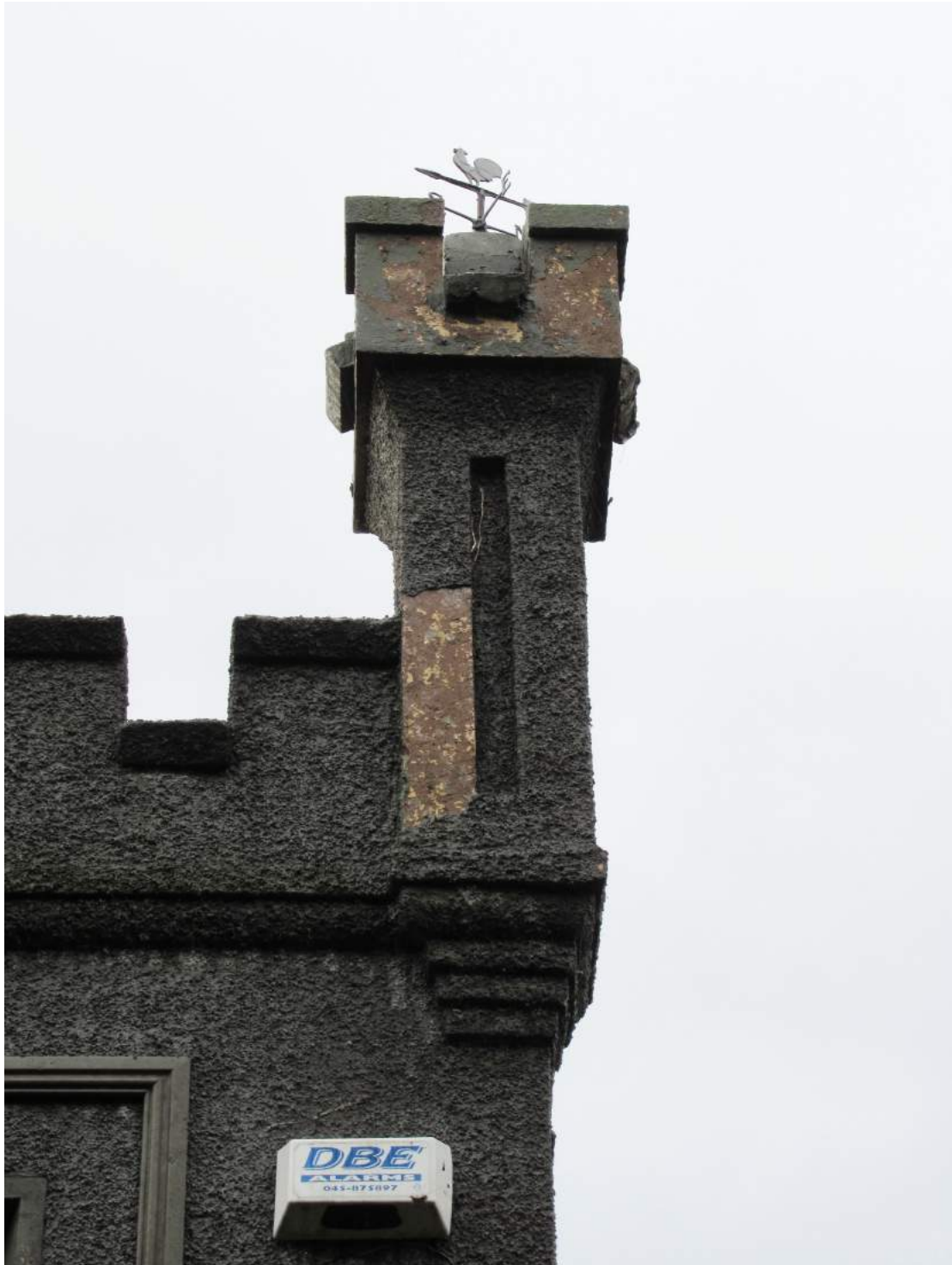
Plate No. 13. Detail view showing one of the rendered masonry corner battlements, on the primary east elevation to Frankfort Castle. This photo clearly shows the original brown coloured patent cement render under the late 20 th century sand and cement dashing. Note the late 20 th century cast sand and cement moulding over the window at the left.
