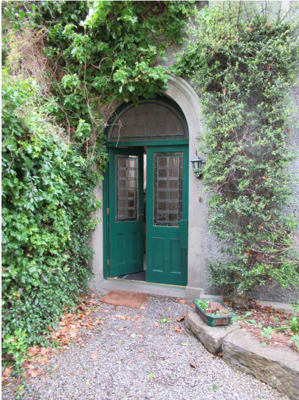
Plate No. 9. Detail view showing the east front door to the northern half of the original house. There is a similar door on the opposite side of the thick hedge at left, leading into the southern half of the original house. Historic Ordnance Maps show a small entry portico or porch attached to the front of the house in this location, probably with a single grand central entrance door.
