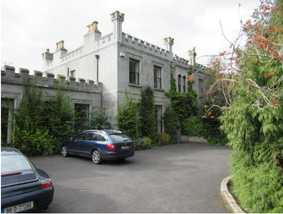
Plate No. 5. View of Frankfort Castle from the south-east. The single storey section at the left is believed to date from ca. 1860, along with most of the two store main structure.
