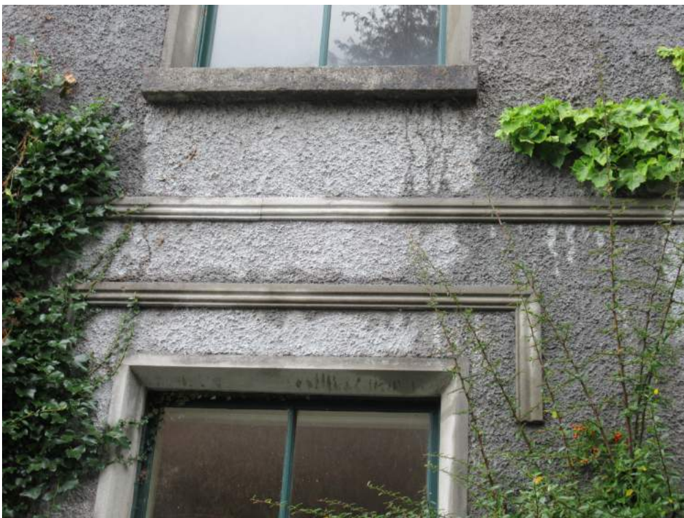
Plate No. 11. Detail view showing some of the windows on the east elevation of the original house. Note the cementitious dashed render, and the precast sand and cement ornament.
