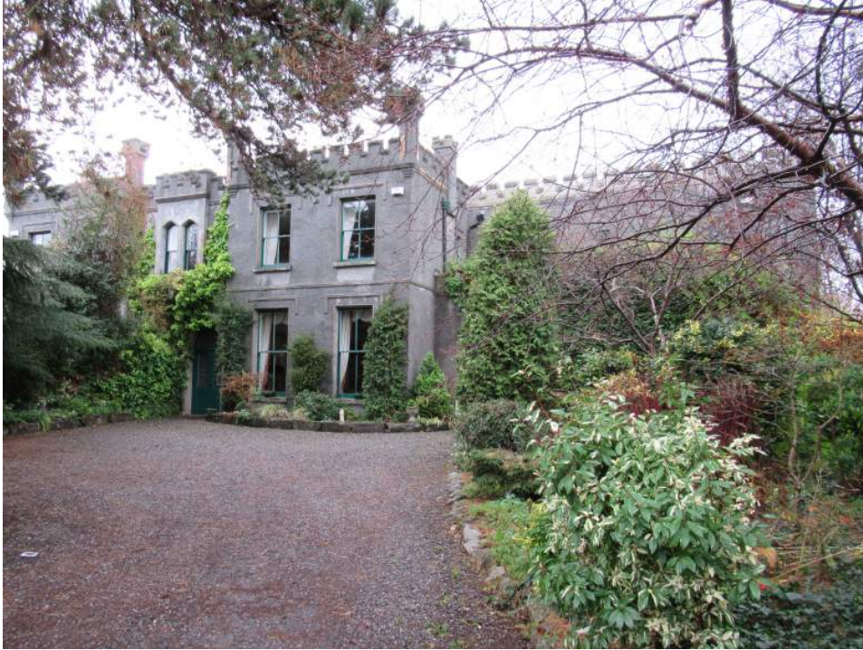
Plate No. 7. View of Frankfort Castle from the north-east, showing the northern end of the structure. The original symmetrical east front can be seen at left, having been subdivided around 1930. The recessed two storey extension at the right dates from the late 20 th century.
