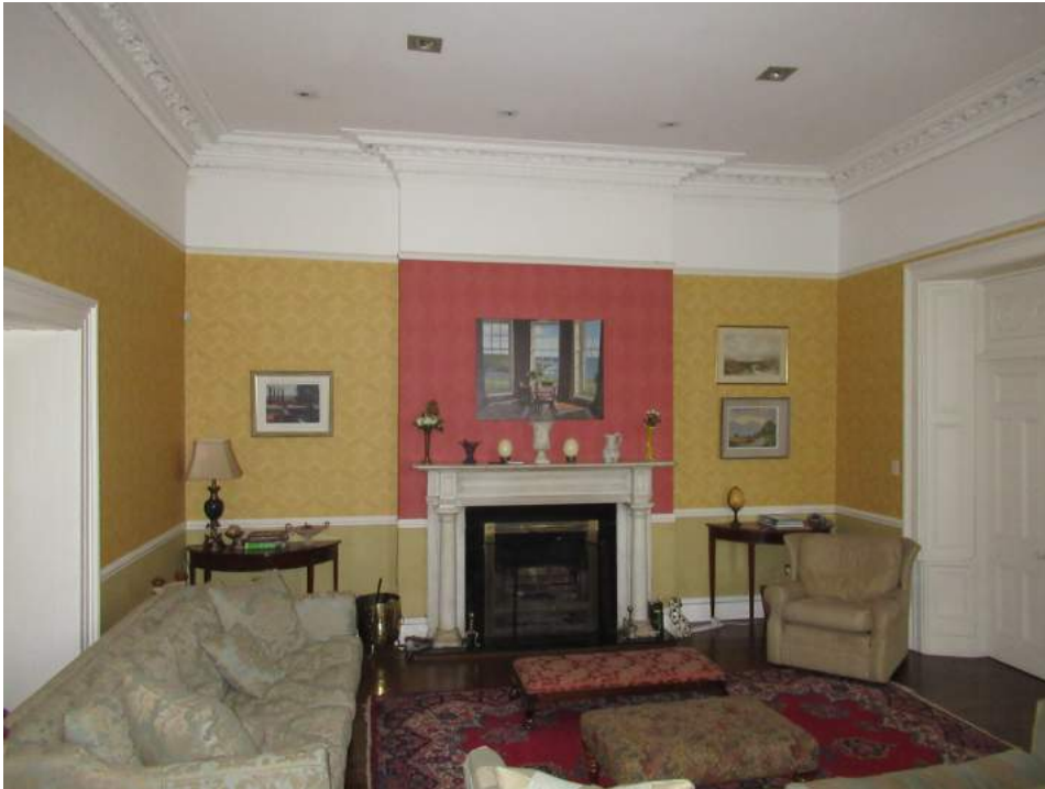
Plate No. 20. Detail intern view showing the sitting room in the northern half of the original house. This room retains mid-19 th century joinery, plaster coving and marble chimneypiece.
